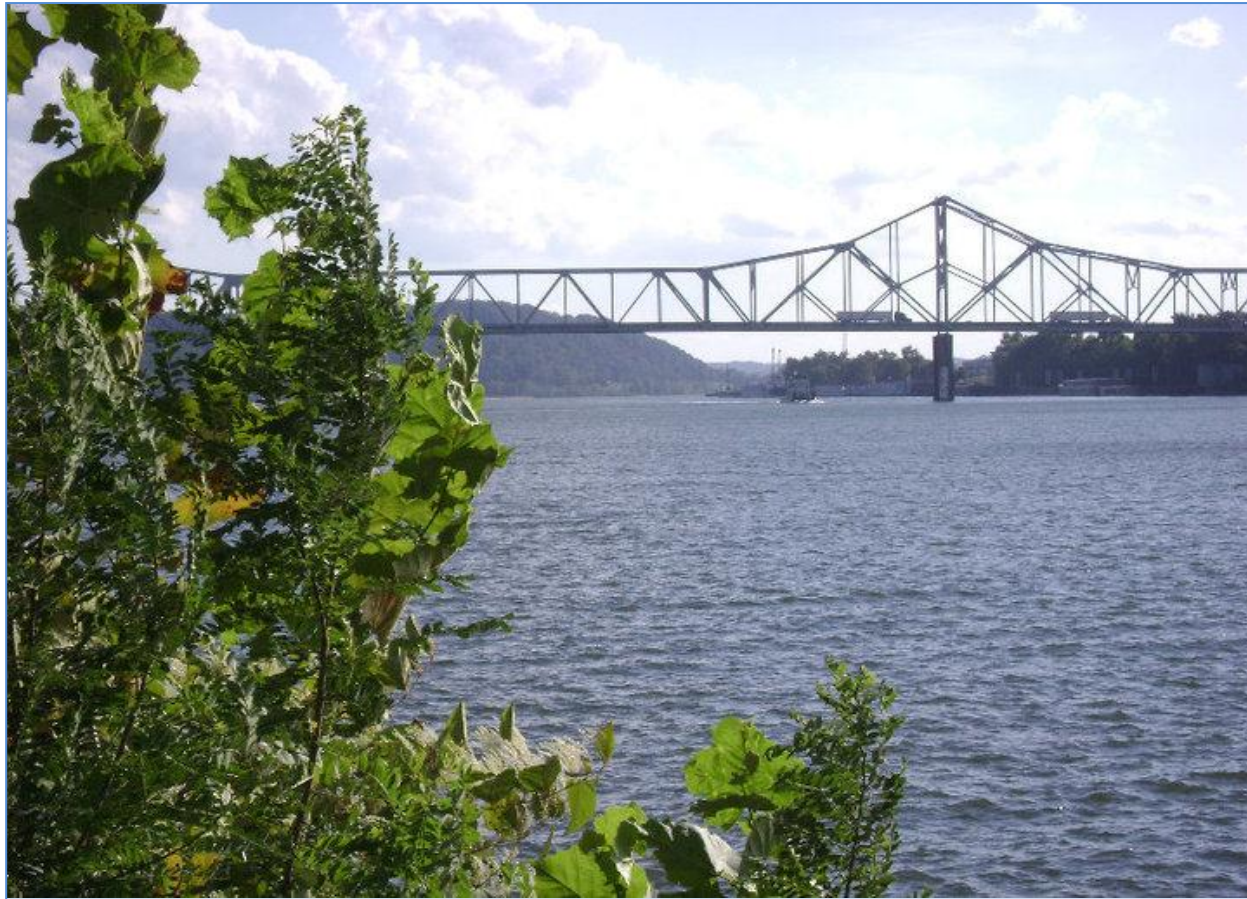
Memorial Silver Bridge at Point Pleasant connecting West Virginia and Ohio
